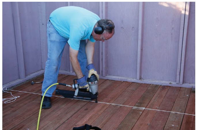
Caption: Eric Dueltgen nails the new decking into place. Credit: Ross Gaunt
