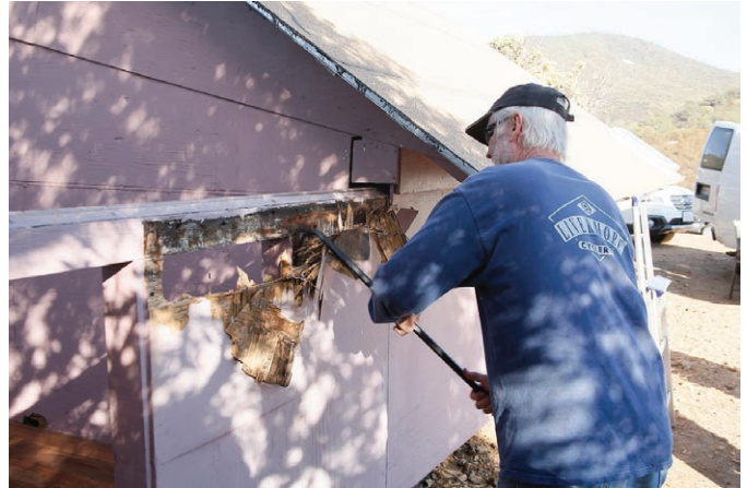
Caption: Rich Combs removes a rotted side panel. Credit: Ross Gaunt
