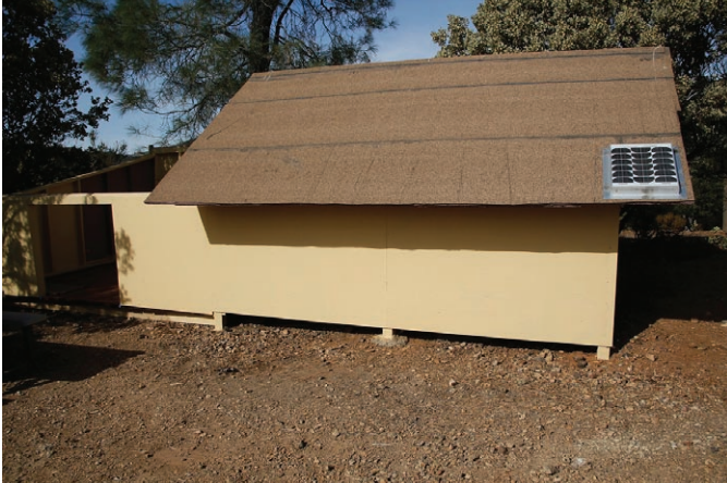
Caption: With a new coat of paint the observatory structure will be protected for years to come. Credit: Ross Gaunt
