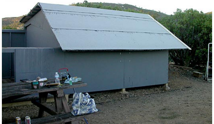
The roof is completed, just before the sun goes down.
